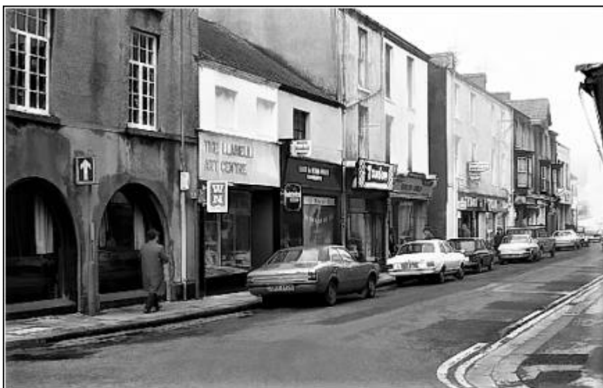
The Llanelli Art Centre after its move from West End to Market Street in the late 1960s
